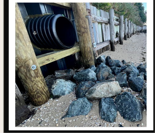
The TOH completed its drainage project at VG which involved bypassing the old clogged pipe and building a stone revetment on the sand to catch flowing water.
