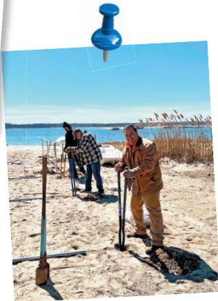
Digging the Holes
