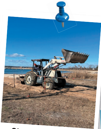
Clearing the Way
