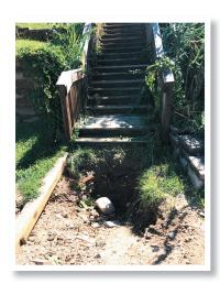
At Valley Grove the water pressure backing up inside the Town drain pipe blew off the metal storm grate. The force of water shooting up through the grate scoured sand at the base of our wall where the pipe runs. With nowhere to go, water at street level pooled then re-directed down POENB stairs, carving out a hole at the base.
